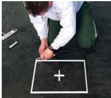
Select point of reference on the roof. Define the positions on the roof for the supports.
