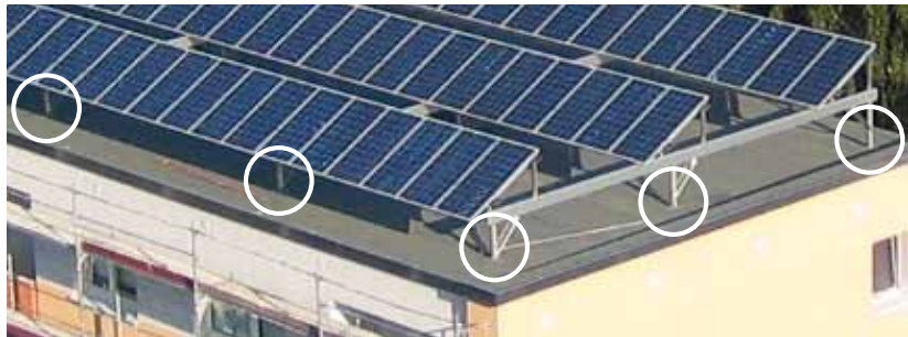
Select point of reference on the roof. Define the positions on the roof for the supports.
